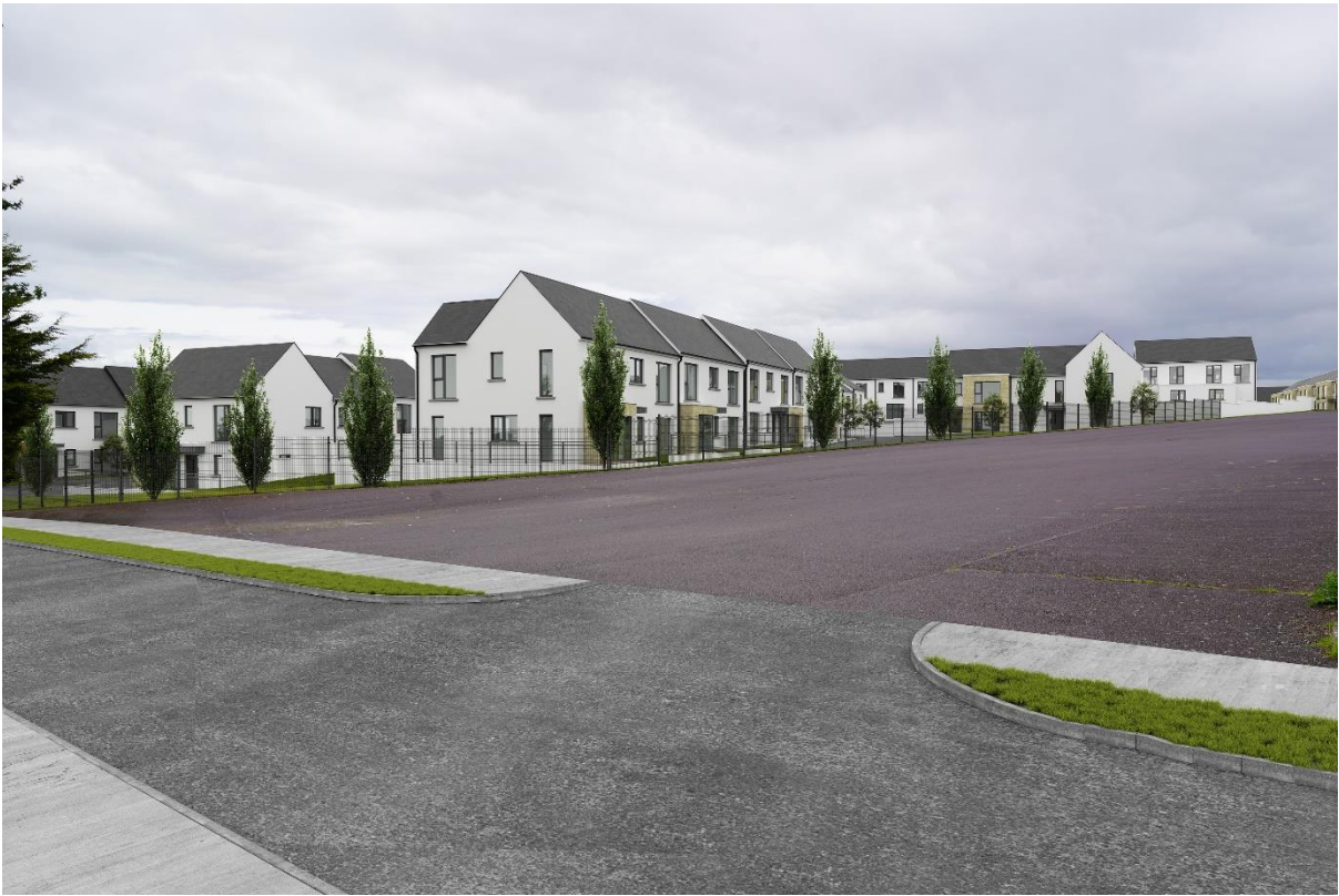
Figure 14: showing the relationship of housing to the existing Delaney's GAA carpark and grounds in the southeast corner of the site.
